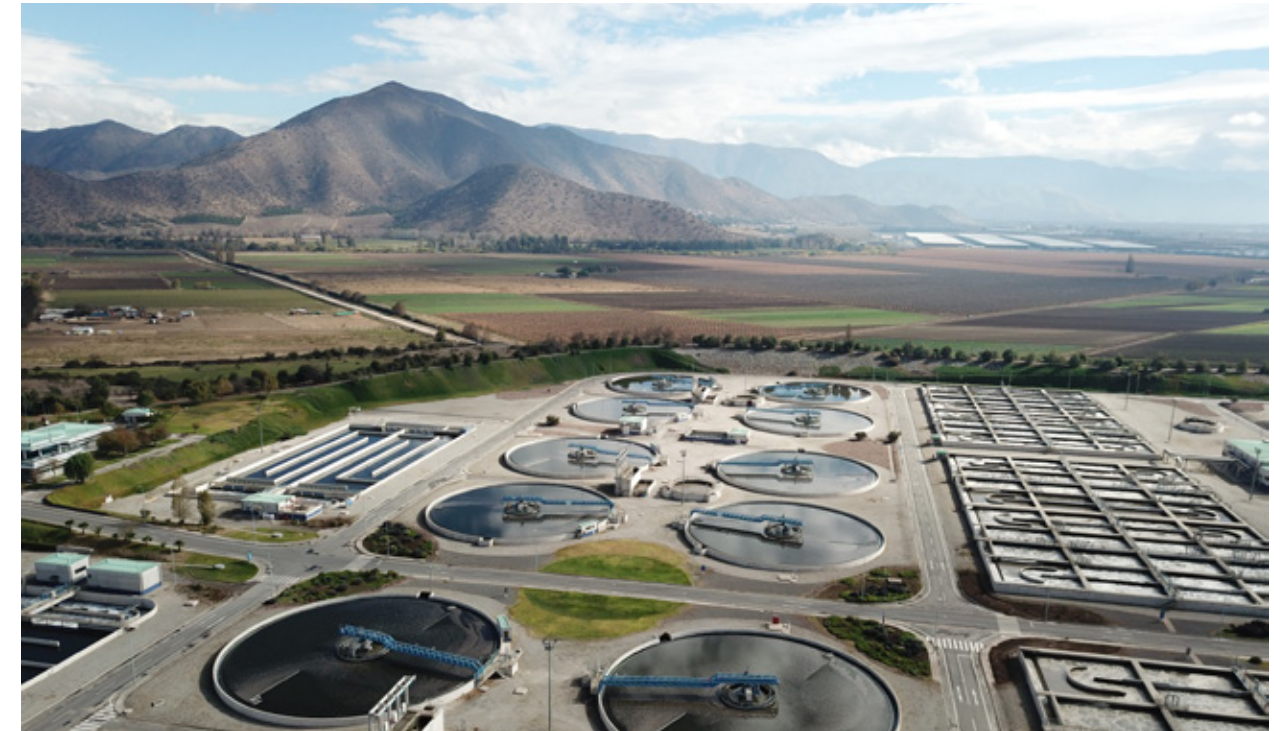
Aguas Andinas' La Farfana wastewater treatment plant as seen from above. The corridor in the top left is where the treated water from the plant gets rechanneled back into the Mapocho River.
