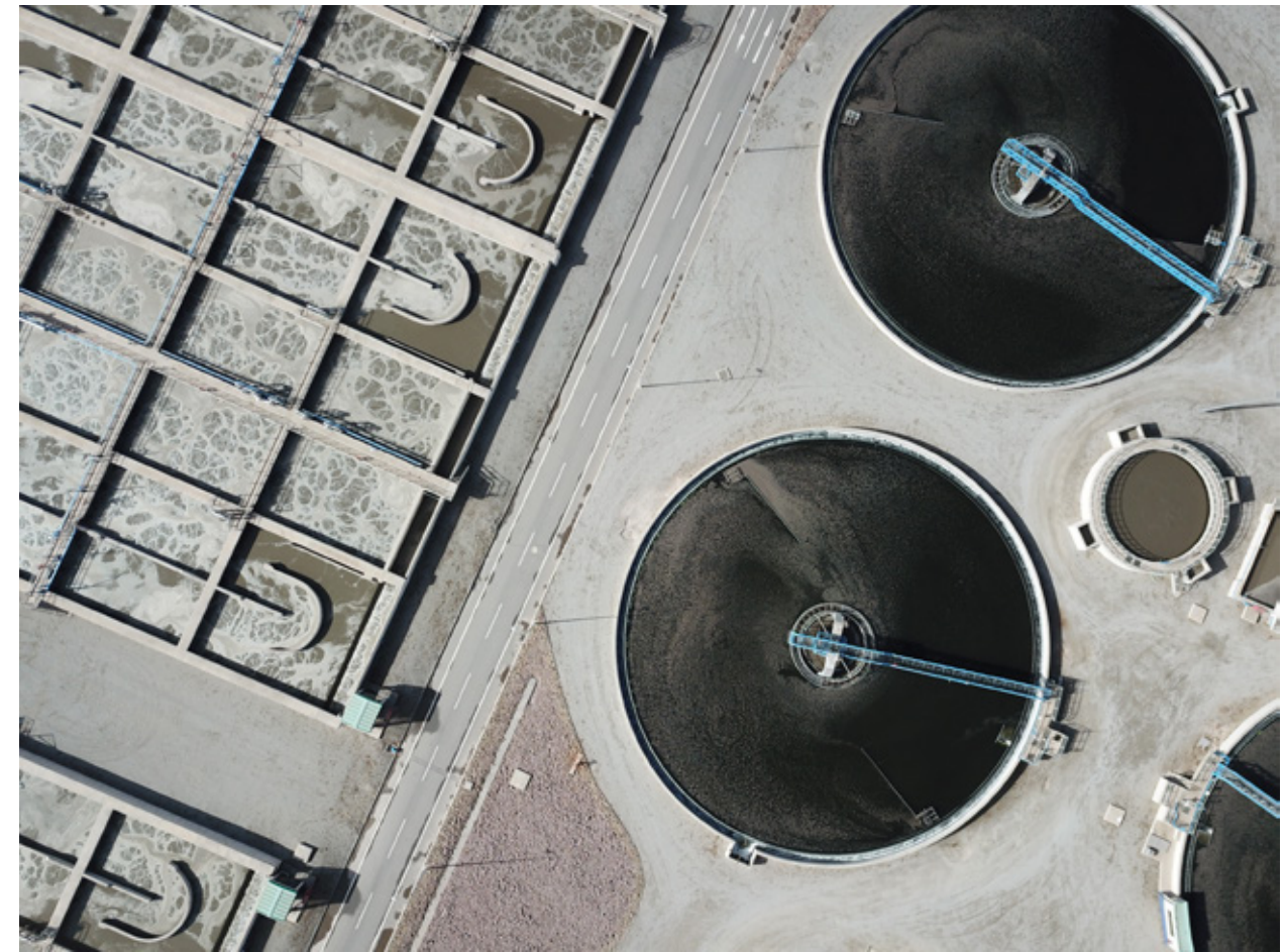
La Farfana's wastewater cleaning mechanics from above.
